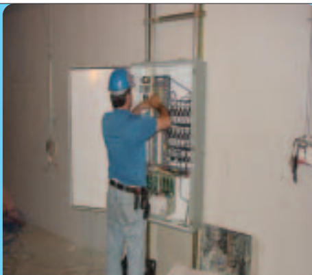
T.E.C. Systems' technicians configure, test, and commission local controls panels throughout the facility.
